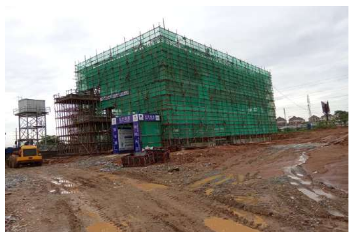
Comprehensive Building at completion of frame structure.
